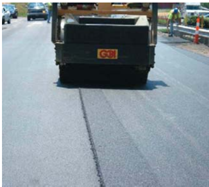
Vibratory compactor passes over an 18-inch-wide section of uncompact material along the joint. Note that the roller pass laps over the cold mat.
